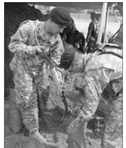
More sandbags are filled by the Soldiers. As of last Wednesday, El Paso city personnel had distributed 80,000 sandbags.
